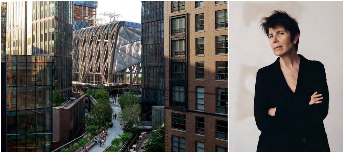
The Shed, an arts center in the Chelsea neighborhood of Manhattan, by Diller Scofidio + Renfro in collaboration with Rockwell Group. Right, Elizabeth Diller. Timothy Schenck; Geordie Wood
